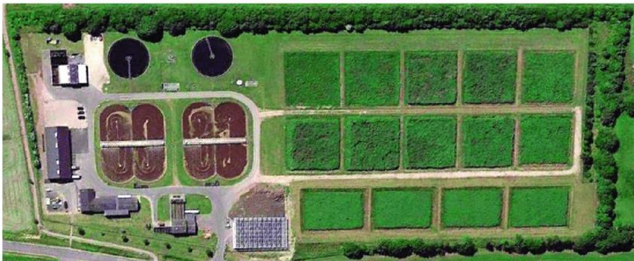
Prilog, Slika 7. Polja za ozemljavanje mulja uz UPOV ( https://www.researchgate.net/figure/Overview-of-a-typical-40-000-person-equivalent-sludge-treatment-reed-bed-system-in_fig1_314028719 )
