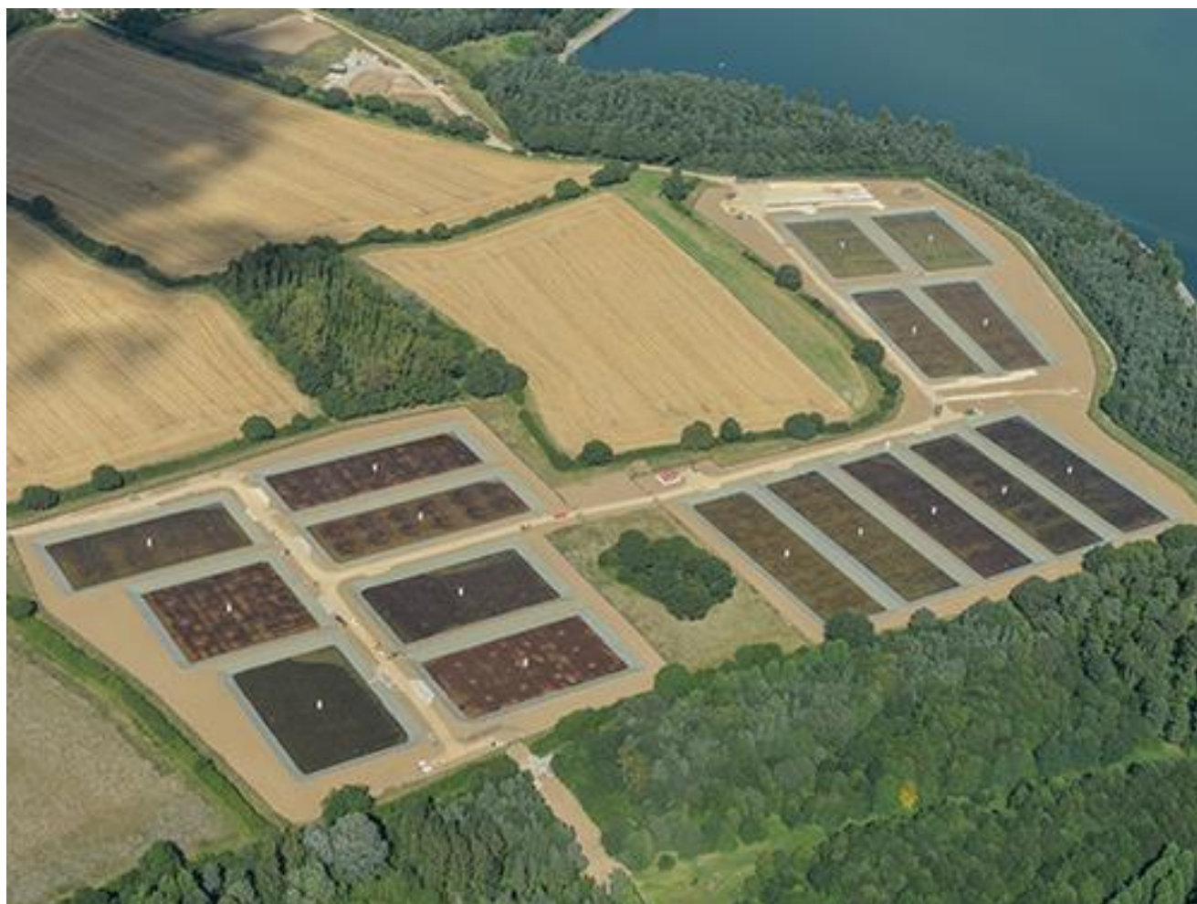
Prilog, Slika 8. Polja za ozemljavanje mulja ( http://waterandcarbon.com.au/project_category/sludge-treatment-reed-beds/ )
